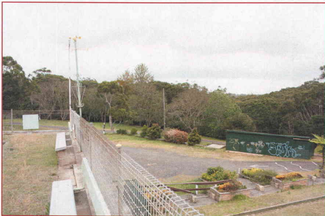
PHOTO 7: Leaning seat indicating settlement
