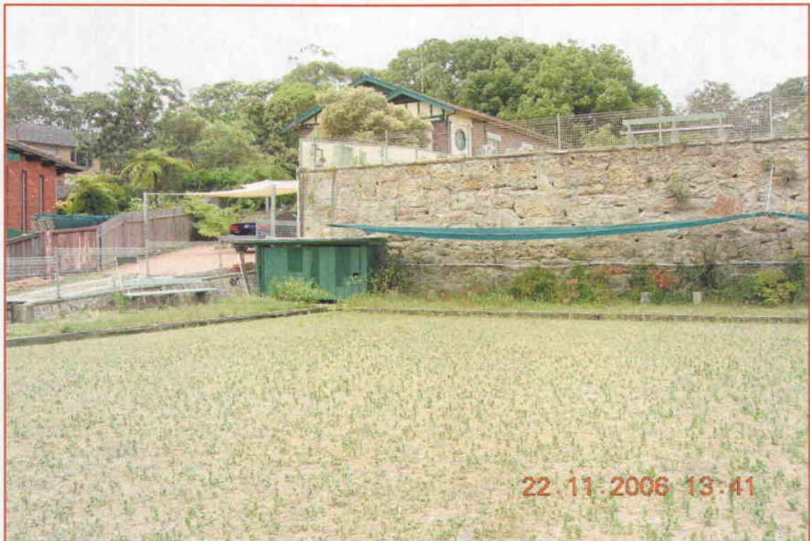
PHOTO 4: Retaining wall between greens
