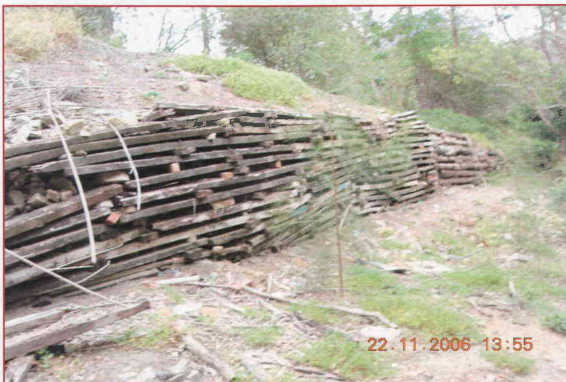
PHOTO 9: Timber crib wall
